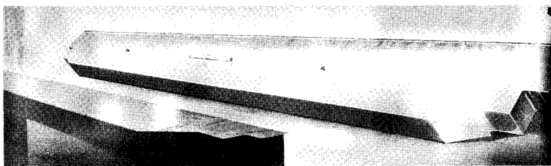
Fig. 9. Welded girder, one ready for cover plate, other in process.
