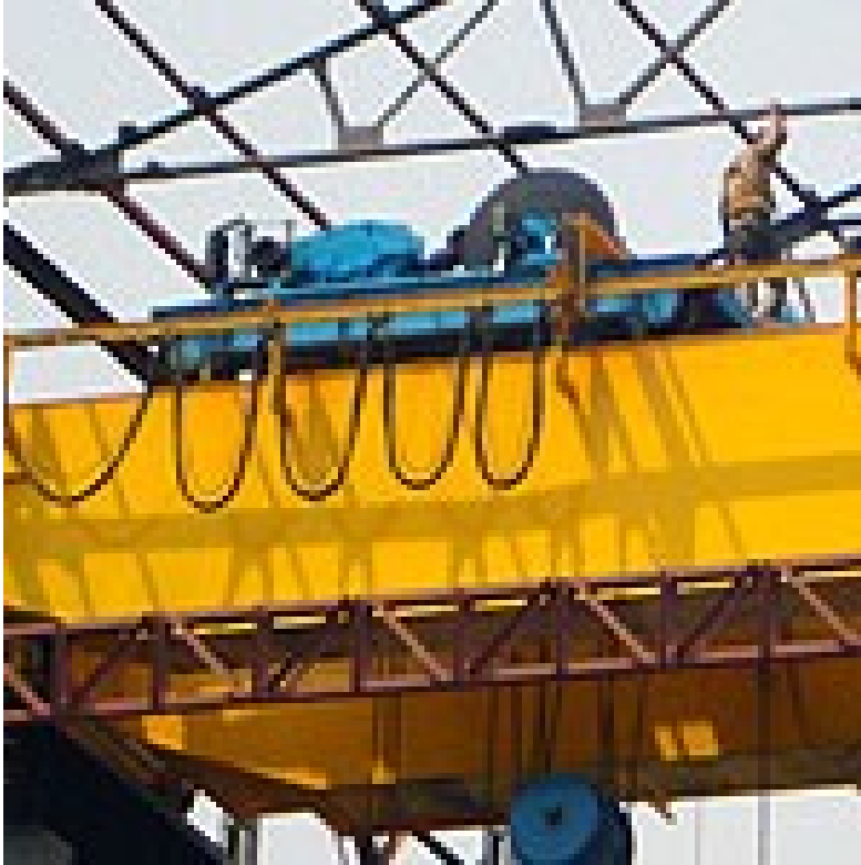
Fig.:- Aerial View of Double Girder E.O.T. Crane.
