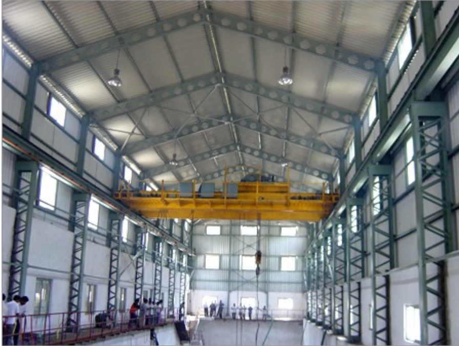
Fig.:- Aerial View of E.O.T. Cranes.
